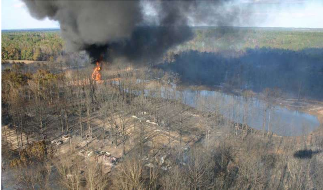
Figure 1. Rupture and explosion of hazardous liquids pipeline, Carmichael, Mississippi, 2007 (source: NTSB).
